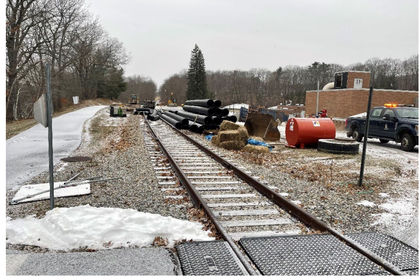
Britt Gully Road crossing, Augusta
