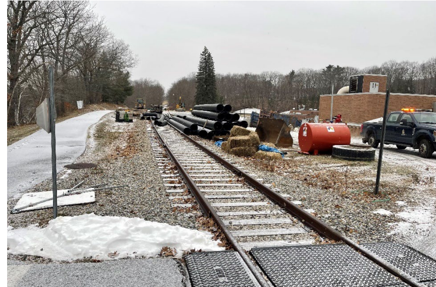
Britt Gully Road crossing, Augusta
