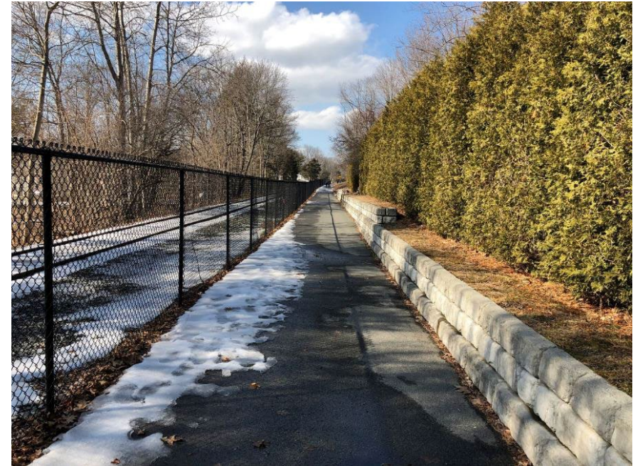
RWT in Ellsworth (with MaineDOT-approved 10.5' offset with fence)
